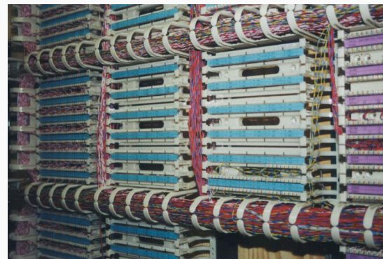
Blocos 110 de 300 pares c/ jumpers
